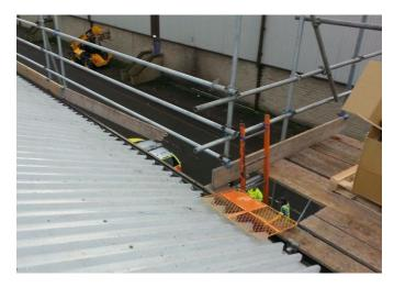
The investigation also revealed that roof lights were present on the roof and that the contractor had failed to take effective measures to prevent workers falling through these fragile surfaces.
