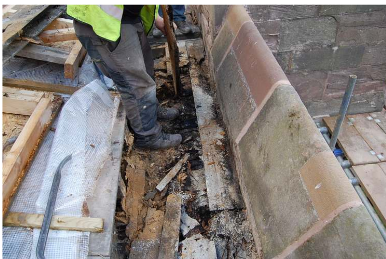
Timber repairs to gutters showing the extent of the decay. James Matthews wrestles with a decayed board.
