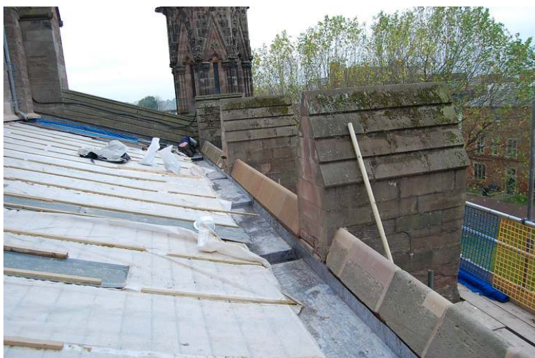
Following timber repairs the parapet gutters are lined with lead.
