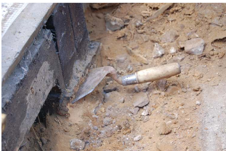
A rather soft truss tie beam bearer.
