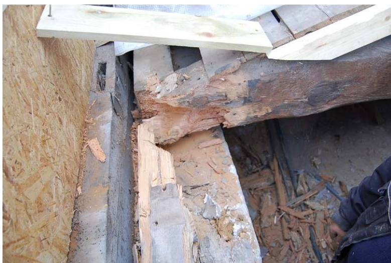
Decayed truss end that required a steel plate.
