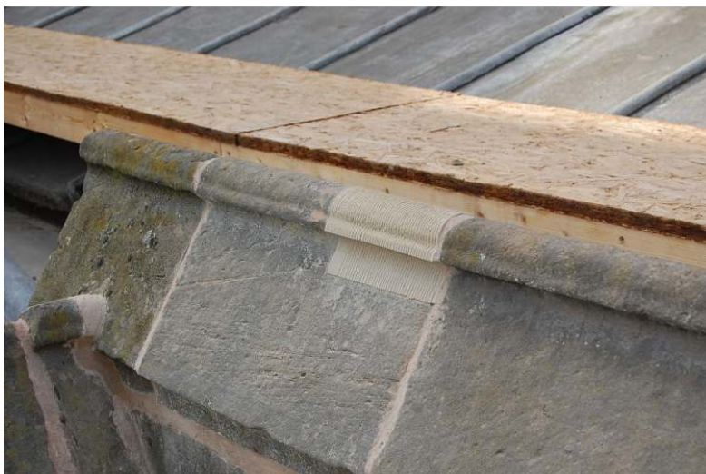
Stone coping with indent repair.
