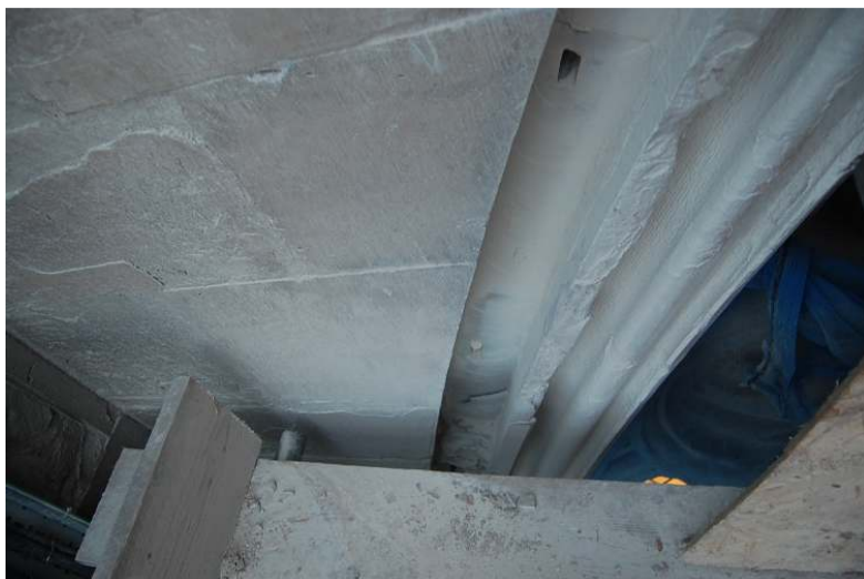
Hood mouldings cut out awaiting replacement.
