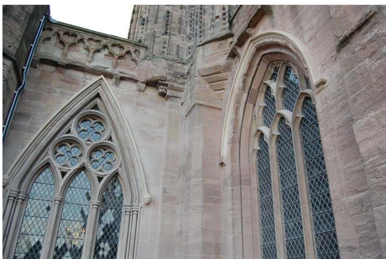
Completed hood mouldings to the North Aisle Clerestory and first bay of the North Transept.
