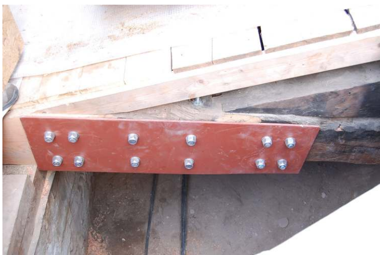
Steel plates both sides of the tie beam hide a new bridled scarf joint but allow as much of the original to remain as possible. Crude but effective.
