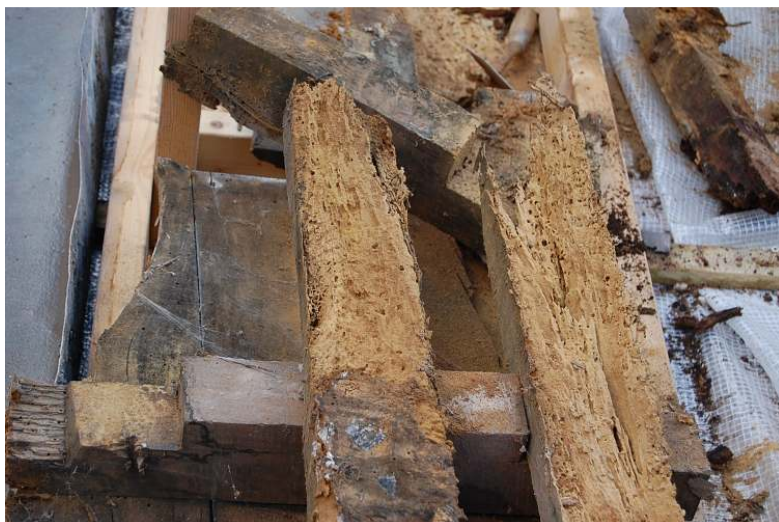
Gutter bearers turned upside down to show the extent of their decay.
