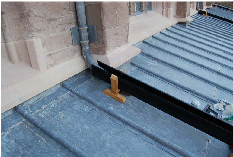
New trough collecting Nave roof rainwater goods.
