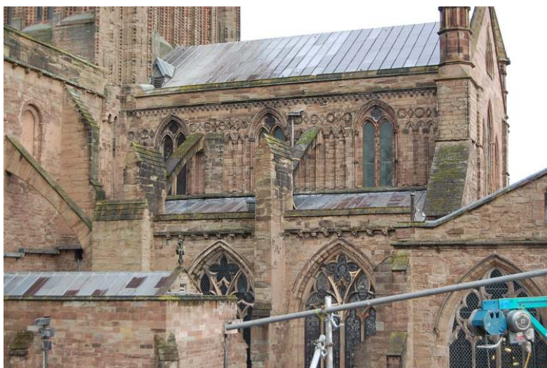
South Quire Aisle patch repairs and part replacement completed.
