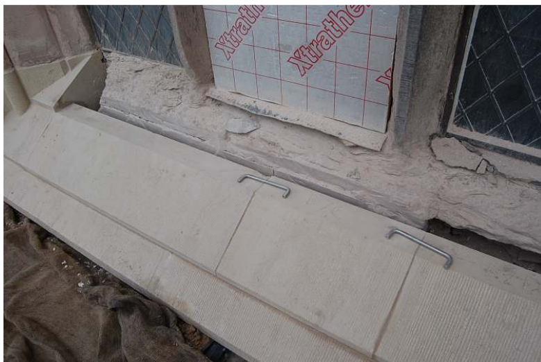
Sill stones with stooling to left jamb and dog cramps awaiting fitting and back grouting.
