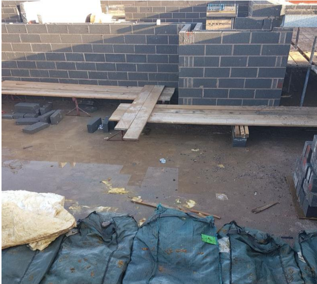
Insufficient working platform?
