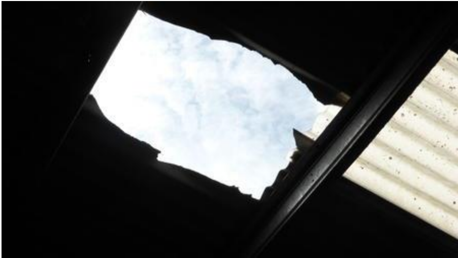
The roof area where the employee fell through
