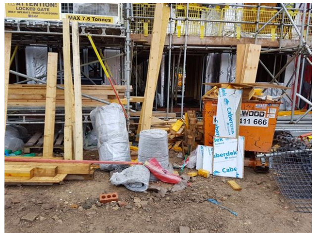
A tidy site is a safe site !!!!
