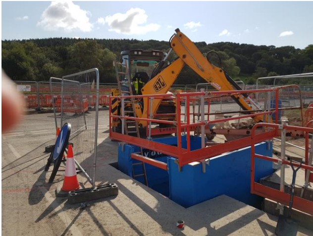
Good example of excavation edge protection
